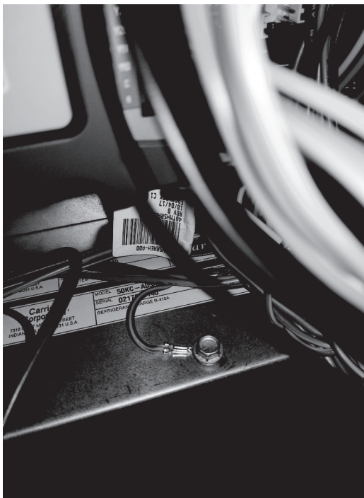
Fig. 12 — Connect Ground Wire From Controller
