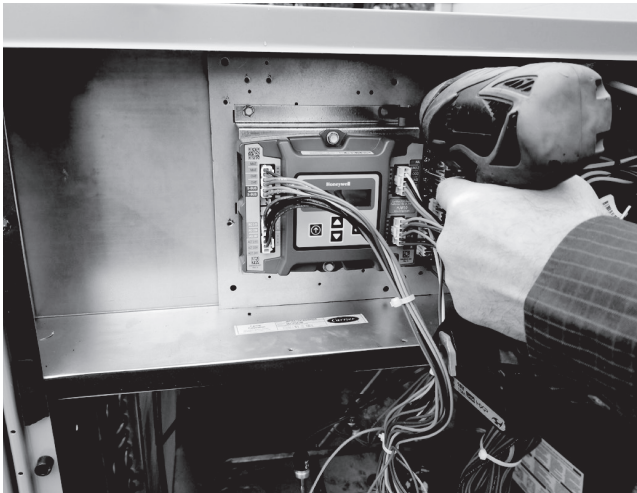
Fig. 7 — Mount Controller Assembly in Unit Control Box (Some control box configurations may differ)
